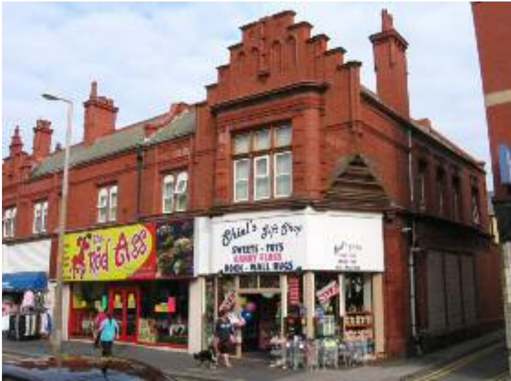
Nos. 16-22 Bond Street, an altered former bank
