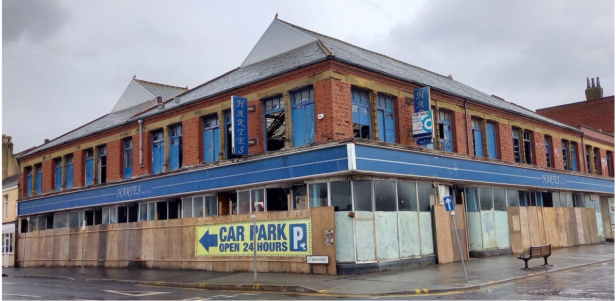
Former Woolworth's store, 7-11 Bond Street
